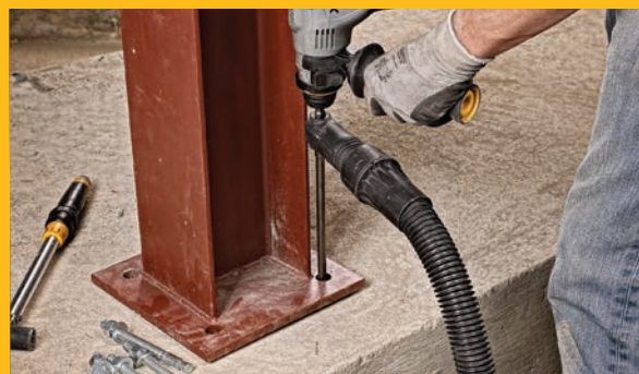
➤ Dust X+™ anchor installation system
